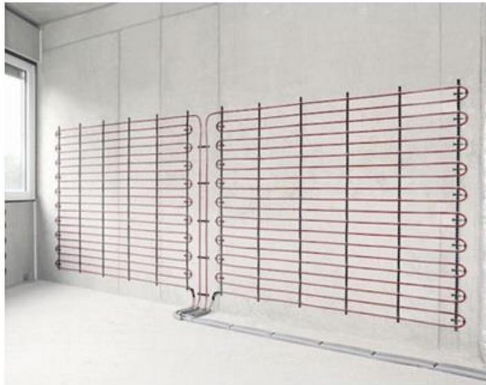
Fig. 4. Sample wall cooling system (Yensis) [8]
